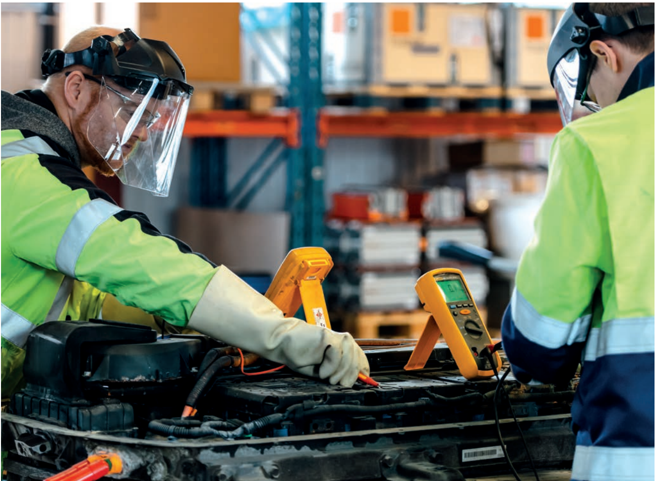
Preparation for reusing batteries. Photo: Batteriretur
