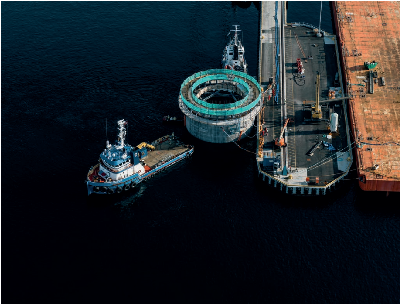
Transportation of concrete elements for Hywind Tampen. Photo: Jan Arne Wold, Equinor
